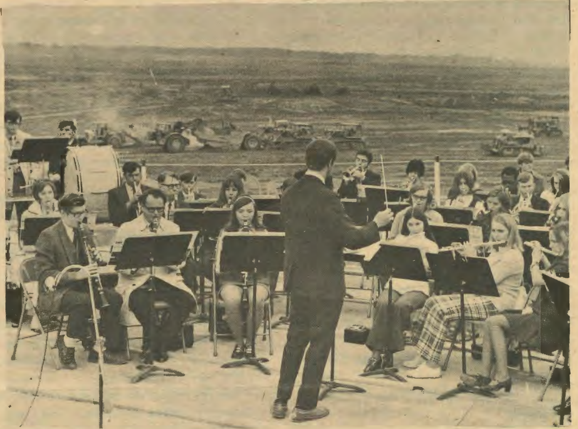
A lot of earth has been moved since RLC construction began. Above, the RLC Community Concert Band plays, under the direction of Bill Hazelbauer, with bulldozers working in the background.
