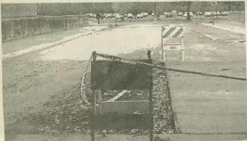
The road under the ACA building should be completed by spring.
