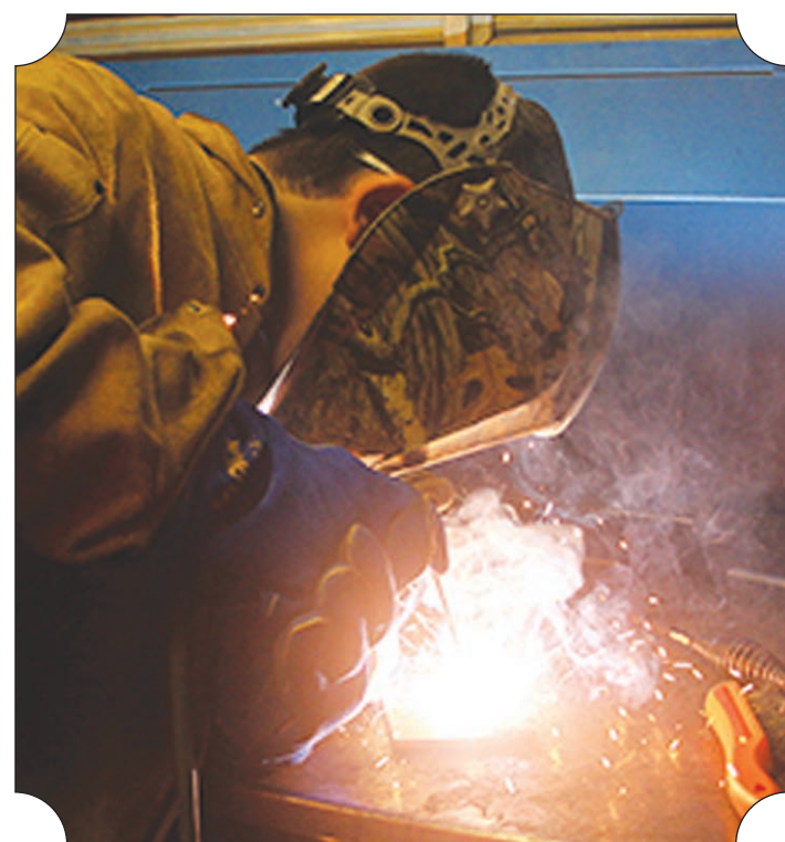
A high school student works in the RLC Welding shop during the 2015 Welding Contest. The top three students win a scholarship to RLC's Welding program. Click on the image for a larger view. (Nathan Wheeler / RLC Public Information)
